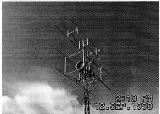
The completed four-band array safely erected
